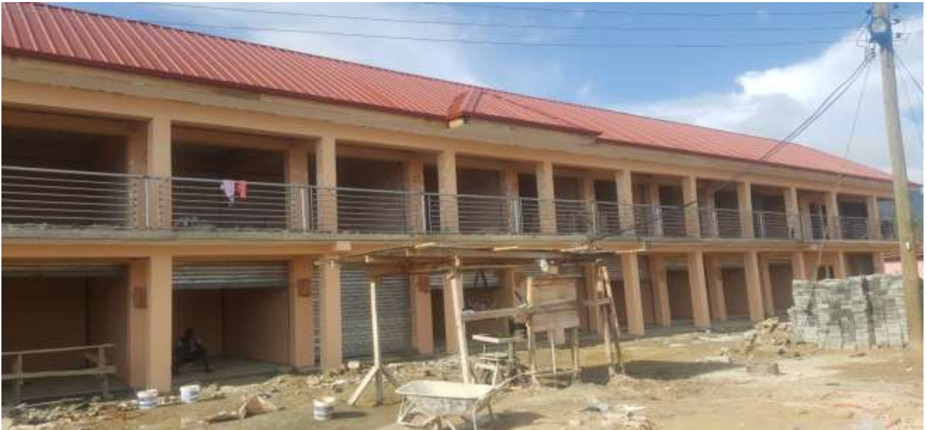
Picture 1: 44 No. 2 storey lockable stores at Nkawkaw Adom
