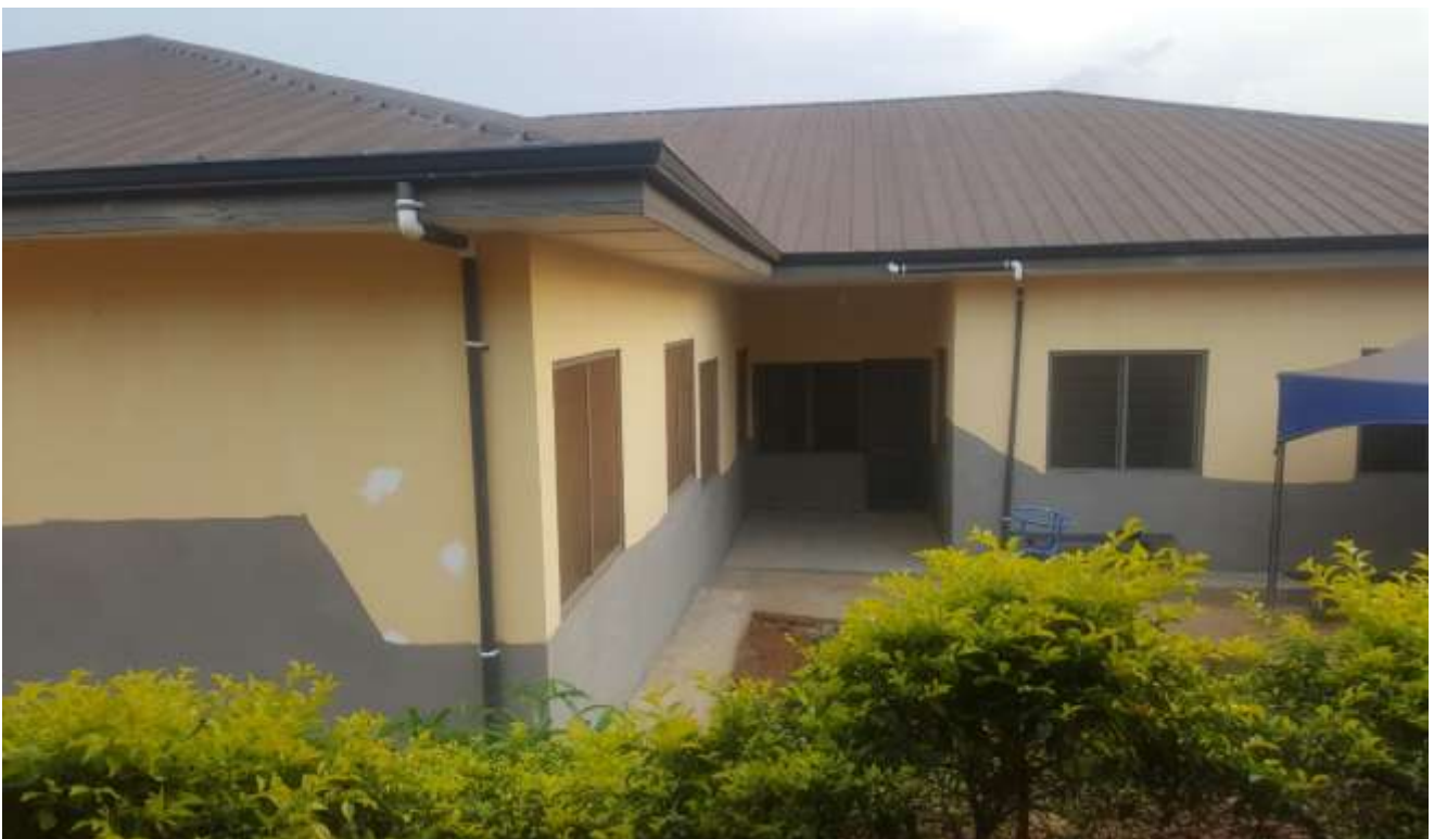
Picture 2: Newly constructed Nkawkaw Health Centre
